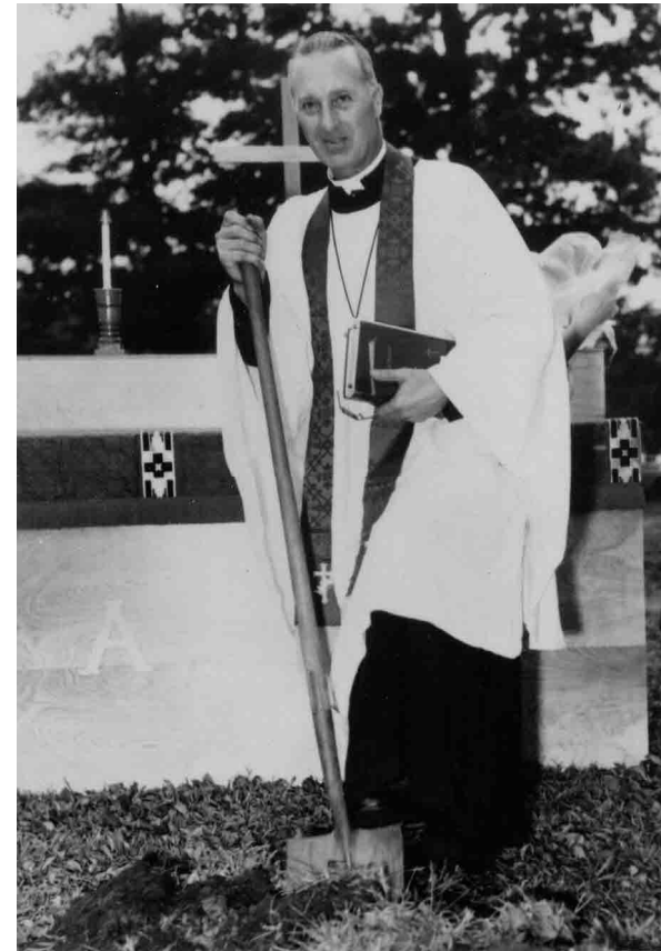
Ground Breaking Ceremony
