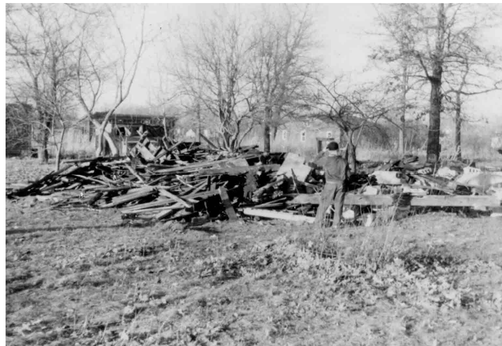
Razed building clean-up
